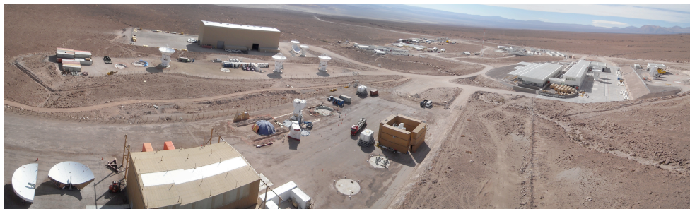
Figure 5: Panorama of the OSF. Left to right: (foreground) European Site Erection Facility (SEF), showing part of one antenna structure; (background) Japanese AEF with three antennas; North American SEF with the large erection hall and two antennas; ALMA base camp; and the the OSF technical building. © ALMA (ESO/NAOJ/NRAO)
