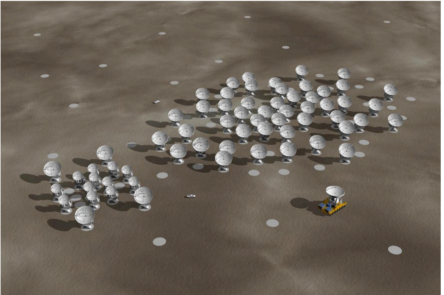
Figure 1: Artists conception of the ALMA compact configuration, with the ACA and “total power” array on the left, and the transporter in the lower right. © ALMA (ESO/NAOJ/NRAO)
