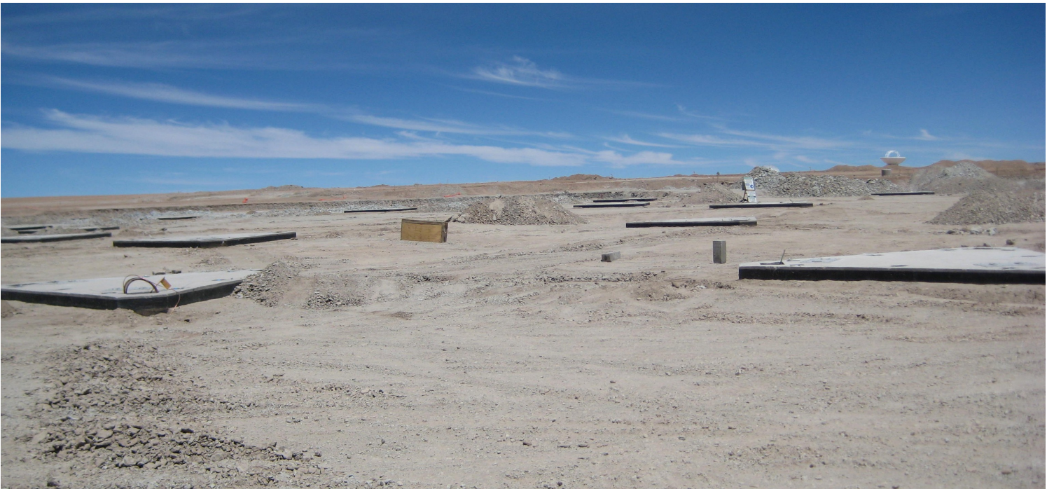
Figure 12: Some of the uncompleted antenna pads of the compact configuration at the AOS. One of the antennas already at the summit can be seen on the horizon.
